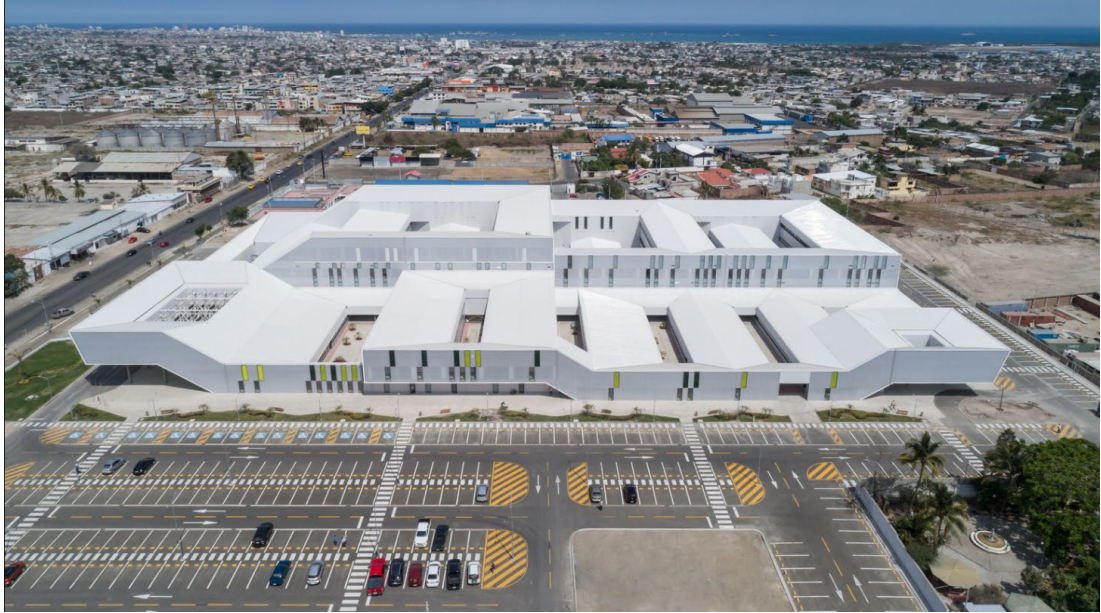
Figura 4. Vista general del Hospital Manta – PMMT, Ecuador
