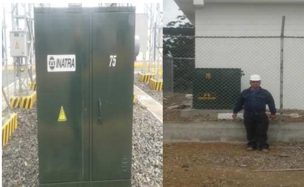
Transformador padmounted
