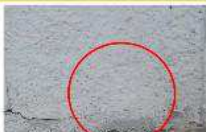
Fig. 1 Erosion
