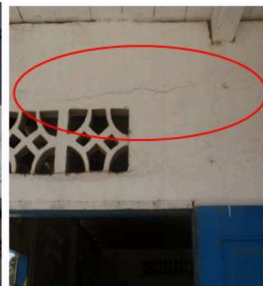
Fig 4. Fisura vertical
