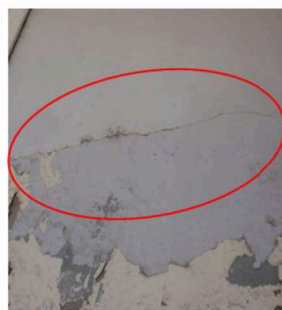
Fig 4. Fisura vertical
