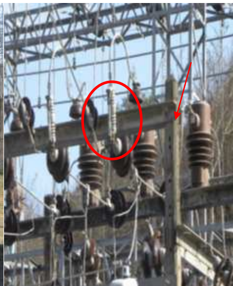
Figura 160. Caja porta fusibles
